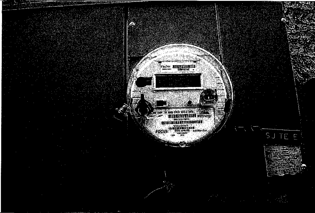
Photo No. 2: Replacement power meters (note mfg. of replacement meter is Landys + Gyr)
